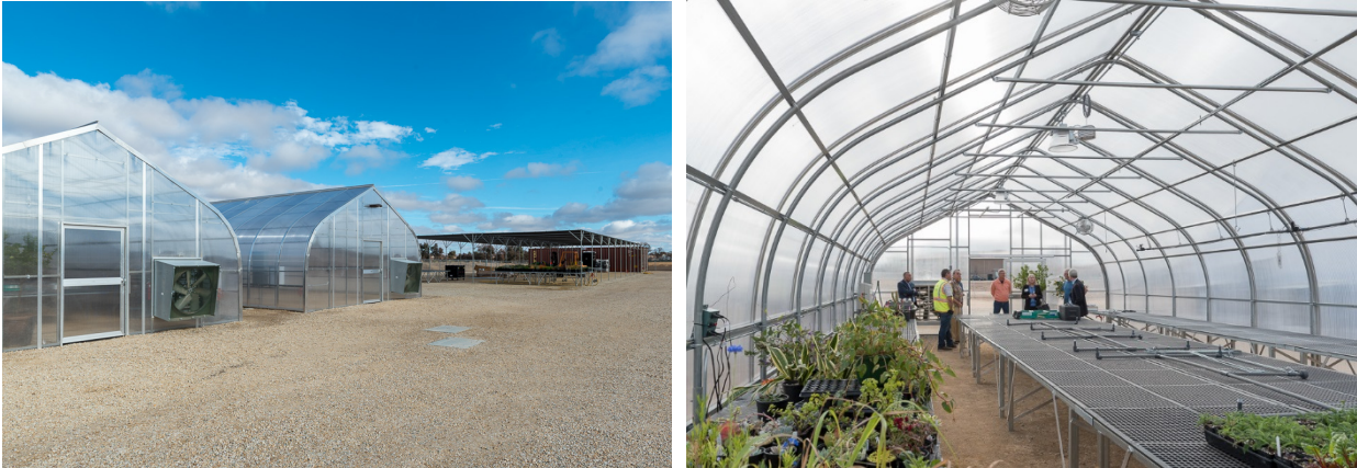
Plant Science Facilities | Greenhouses & Prep for Raised Beds | Greenhouse Interior
